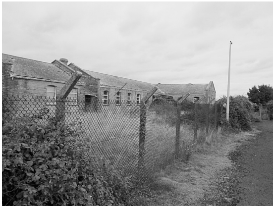
Figure 10. Remains of Somerton Receiving Station, property of South Western Electricity Plc. (Author, 8.18.2018)
