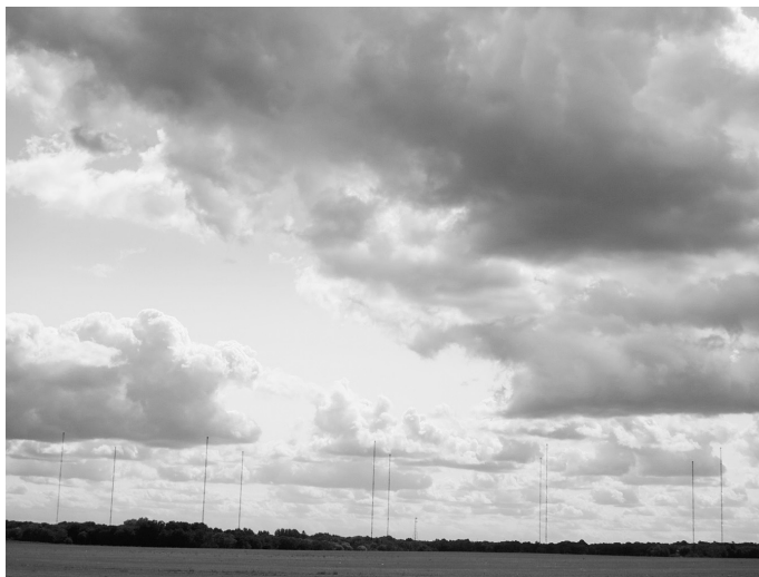
Figure 12. General view of Sainte-Assise Transmitting Station, with ten towers (Author, 8.25.2018)
